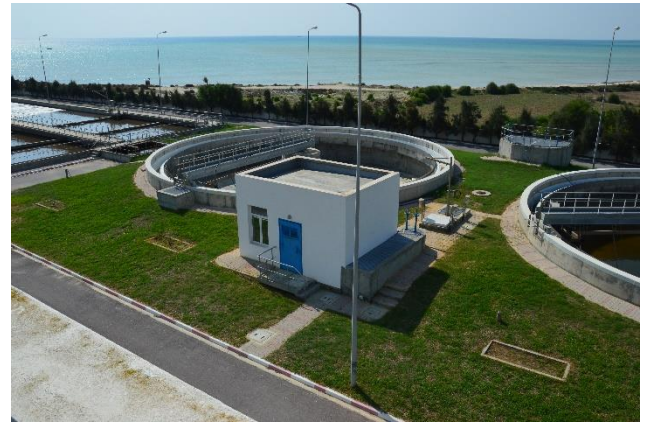
Wastewater treatment plant in Nabeul
